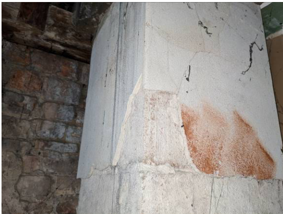
Foto 9: P3.2 - MP Putz Schornstein - Haus 1 - 1.OG - Putz Schornstein
